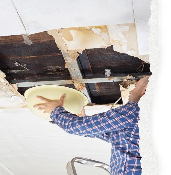
6. Civil - Leaking pipes, drip trays or AC drains leaking constantly overtime and being hidden within the ceiling voids the first you know is when the ceiling falls
